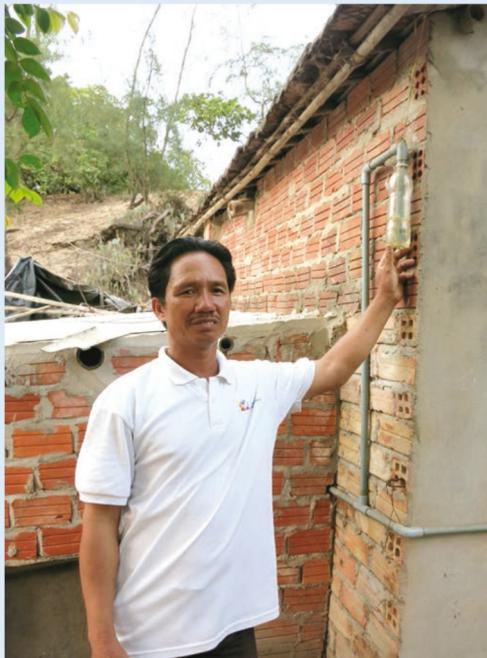
*Thong's biogas pressure gauge measures gas pressure in the tank. Once released, the biogas produces 5-6 hours of fuel for cooking. Photo: Save the children.*
